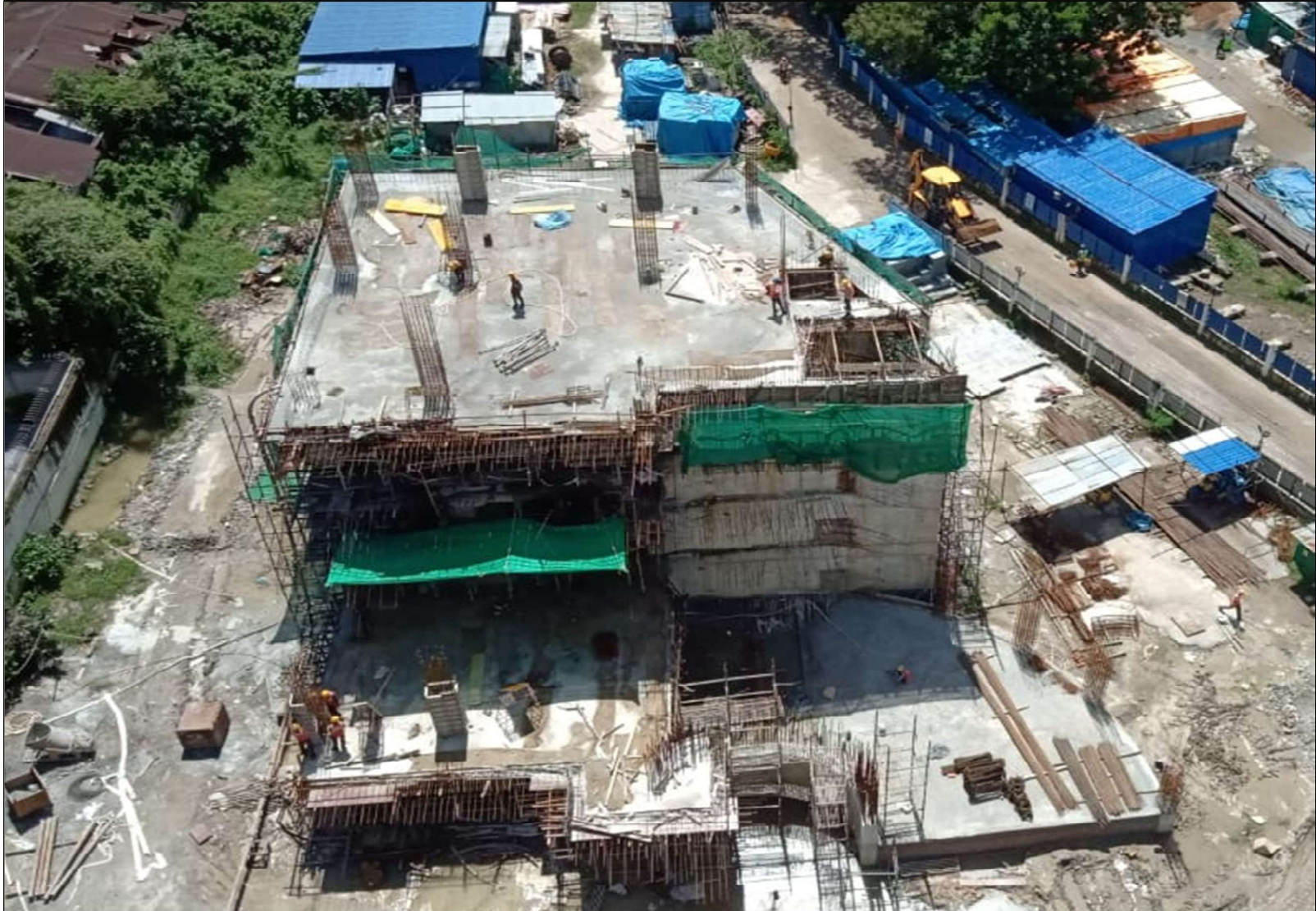
STP area works under progress
