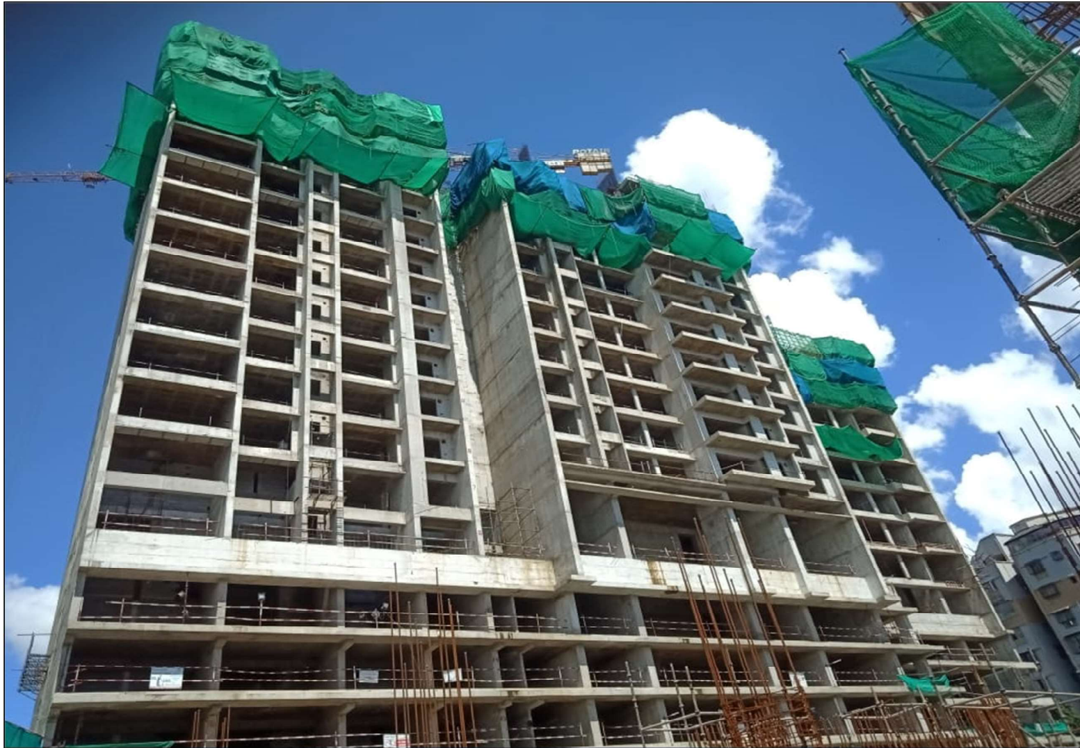
Tower area Shear Walls & Slab under progress
