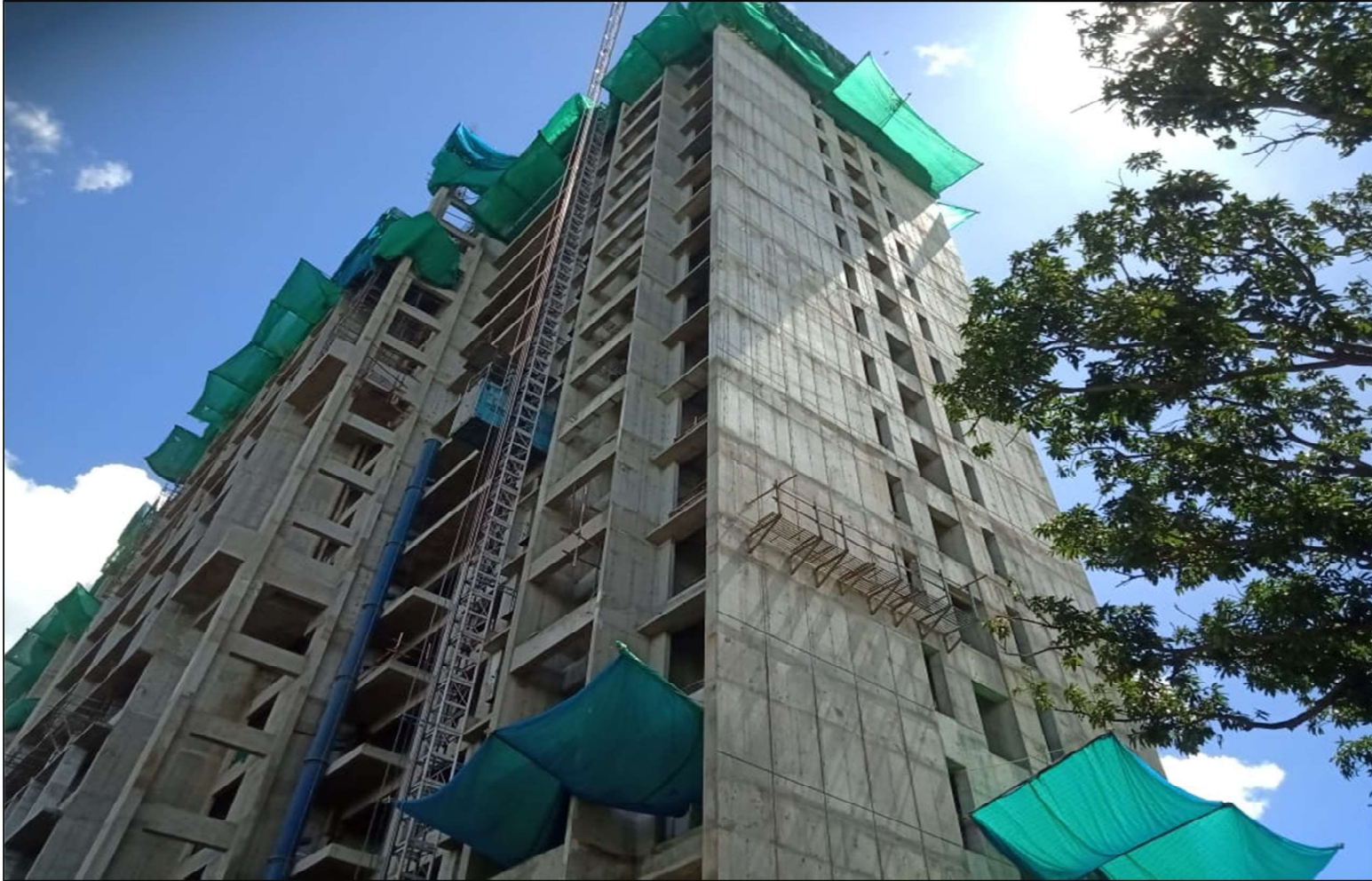
Tower area Shear Walls & Slab under progress
