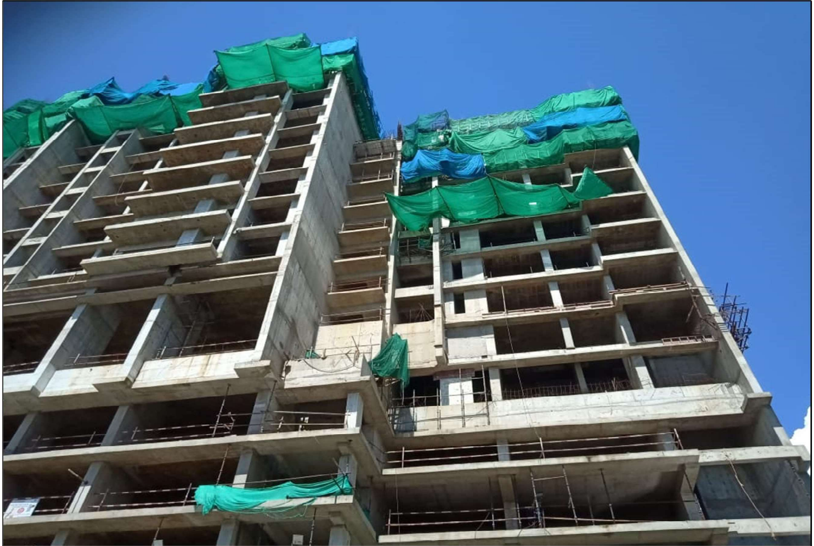
Tower area Shear Walls & Slab under progress
